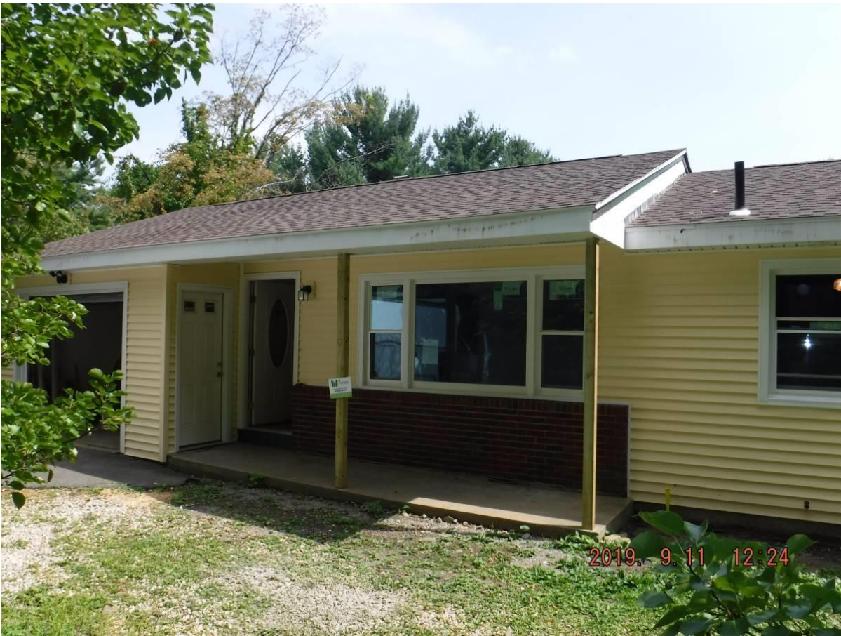
870 East St, Lenox MA - Representative exterior photos showing new roof windows and siding.
