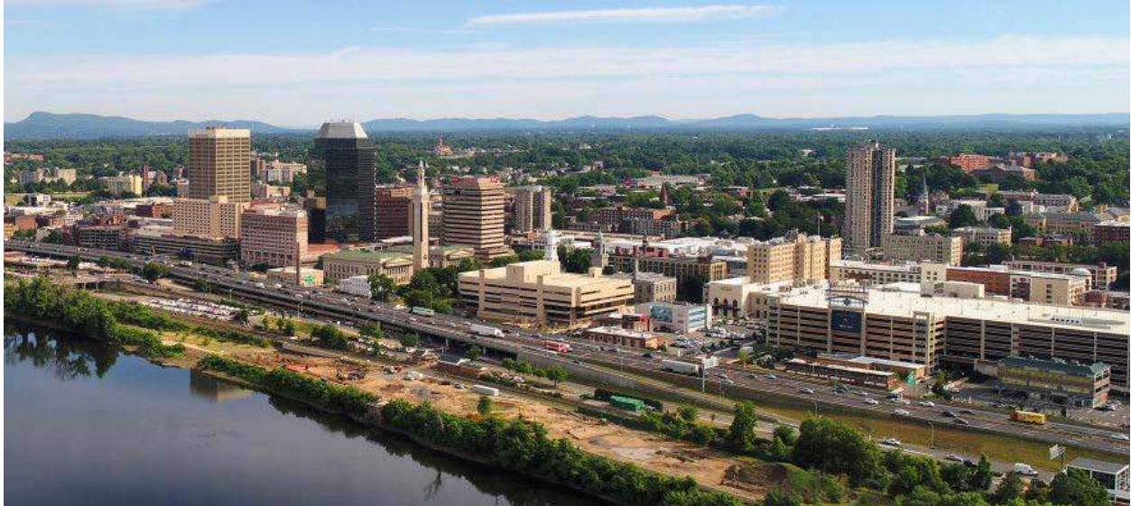
Riverfront Park, under construction 2018
