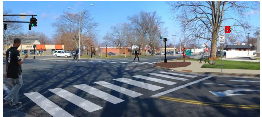
Trail Crossing at Intersection - After
