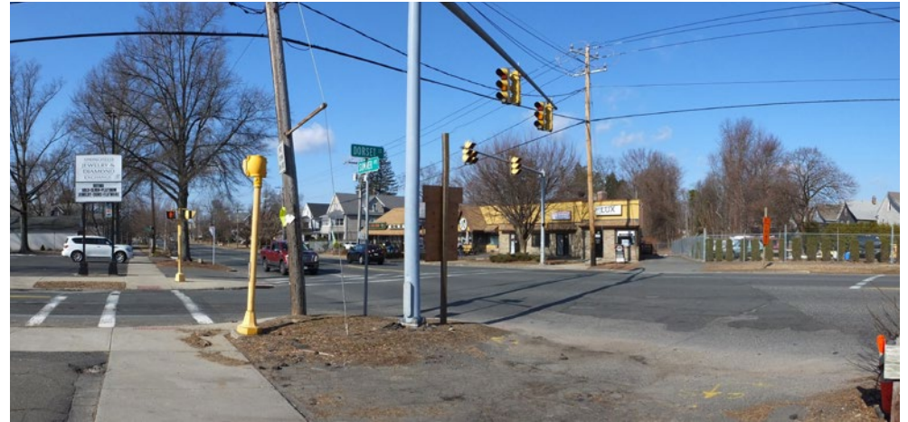
Trail Crossing at Intersection - Before
