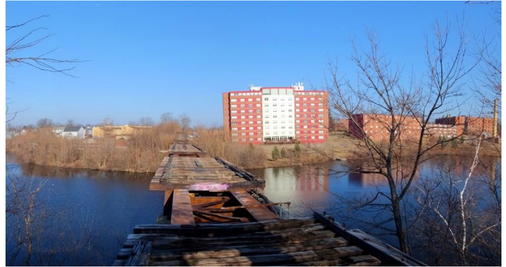
Trail Across Bridge - Before
